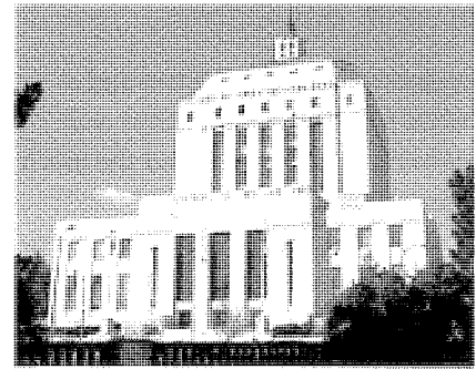
The Alameda County Courthouse is one of 50 county facilities receiving a lighting upgrade. The project is expected to save the county hundreds of thousands of dollars annually in electricity consumption. (Photo courtesy of Alameda County)
