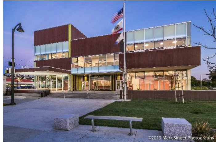
REACH Ashland Youth Center 2013 | LEED Platinum
