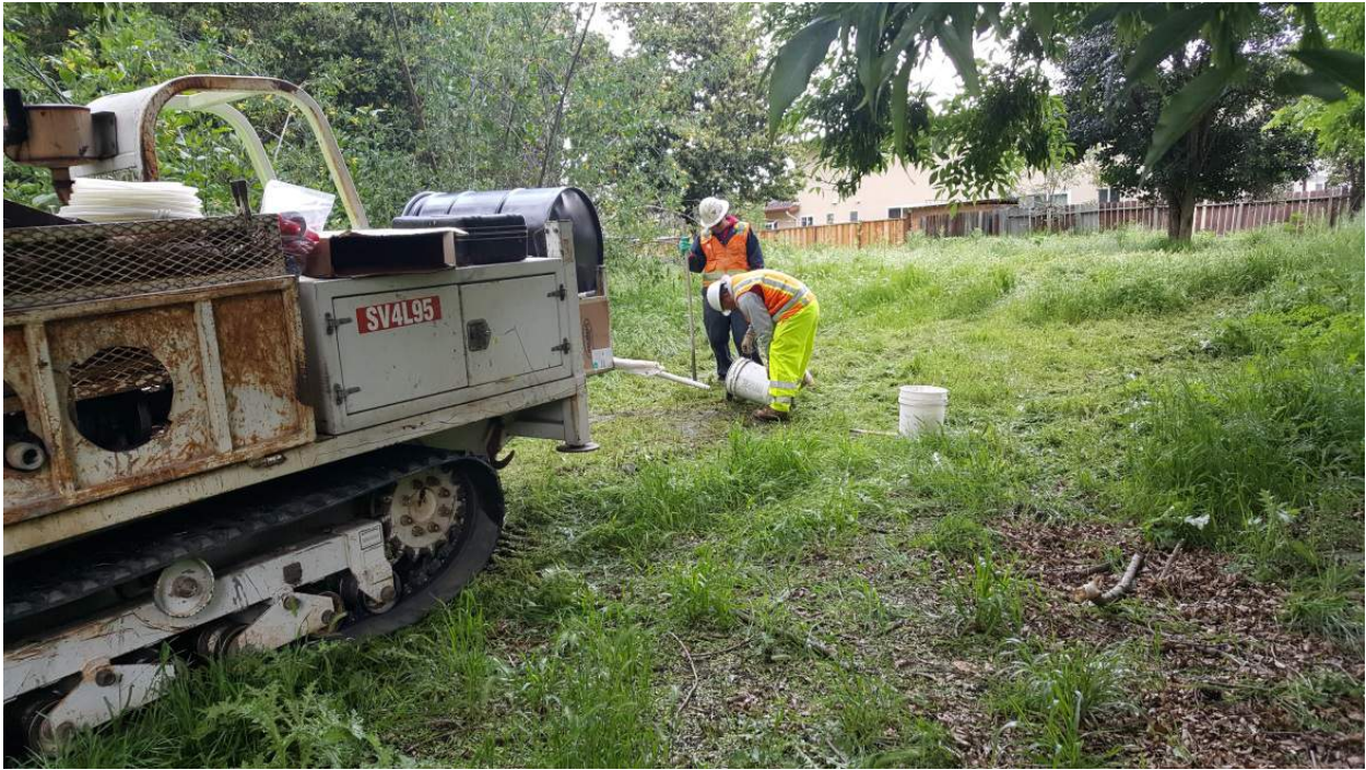
Photo 10: View of bentonite slurry being poured into SB-4, looking northeast.
