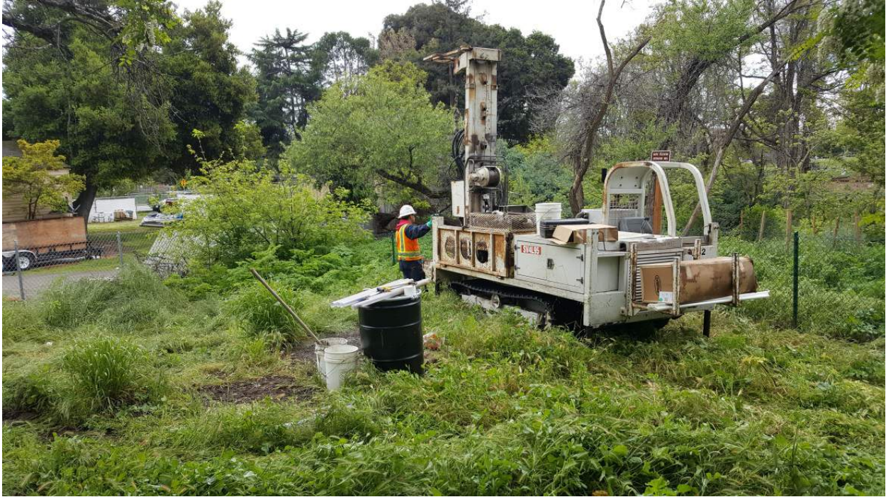
Photo 5: View of SB-2 advancement in progress, looking southwest.
