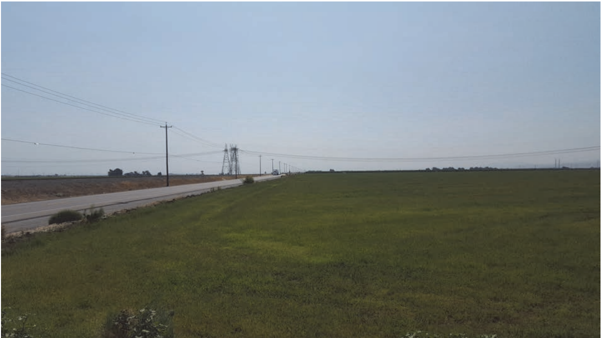
d. View from Byron-Bethany Road at Mountain House Road, looking southeast, showing the site's frontage along Byron-Bethany Road. A set of railroad tracks owned by the Southern Pacific Railroad can be seen on the berm that parallels the left side of Byron-Bethany Road. In the distance, at the end of the flat field, the orchard trees located on the parcel that borders the project site to the south and east are visible.
