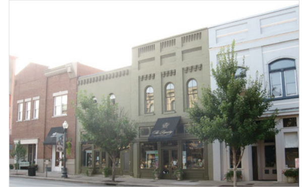
These buildings use brick and other high quality materials that convey a sense of permanence. (Guideline E-6)
