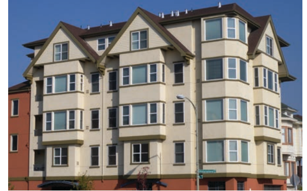
This project uses too many different window designs (different bay window styles, smaller windows are not consistent) which results in an inharmonious facade. (Guideline E-34)
