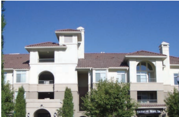
The variable roof elements break the building masses into smaller units. (Guideline E-29)
