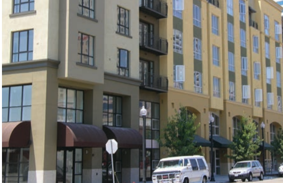
Although this project incorporates several colors into its facade, it does so successfully as the colors are harmonious with each other. (Guideline E-14)
