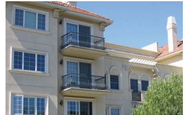
Although the windows on this facade differ in shape and size, the consistent use of trim style and windows with similarly space mullions help create a consistent look. (Guideline E-34)
