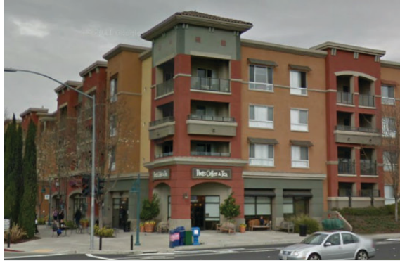
The corner of this building is marked with an architectural element, which provides visual orientation from major commercial arterials. (Guideline C-7)
