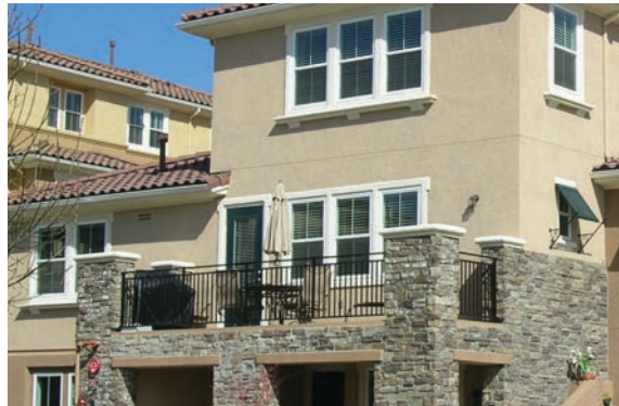
This balcony is dimensioned where there is room for a table and chairs where residents can sit outside. (Guideline K-9)
